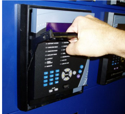
Figure 3-6: Rotate Handle to Stop Position
