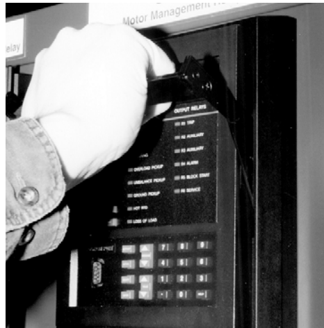
Figure 2-7: ROTATE HANDLE TO STOP POSITION
